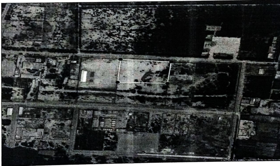
DAMAN FLOUR MILL PRIVATE LIMITED, D. I. KHAN ECONOMIC ZONE DISTRICT D. I. KHAN
